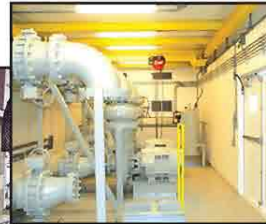
Mechanical and electrical equipment mounted to the steel base and to the sidewalls
