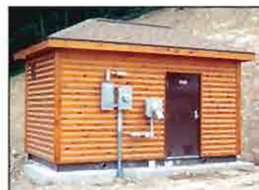
Wood Siding with a Shingled, Hip Roof.
