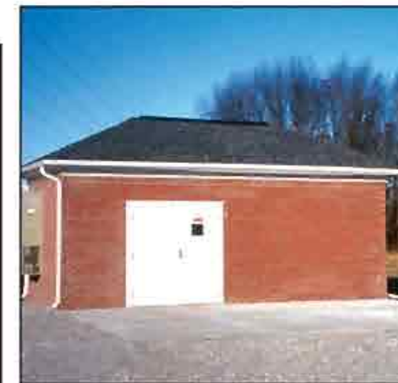
Field Installed Brick with Hip Roof with Fiberglass Asphalt Shingles.
